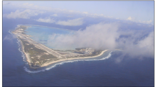
FIGURE 24. HA11 cable landing and CRF.
